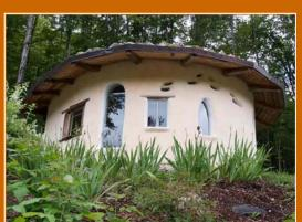
"The Folly" – Art studio built by previous Yestermorrow students. The building is made of cob (a mixture of clay, sand, water and straw) and wood. It also has a green roof covered with vegetation.
