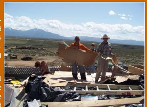
Roof isolation with cardboard (Taos)
