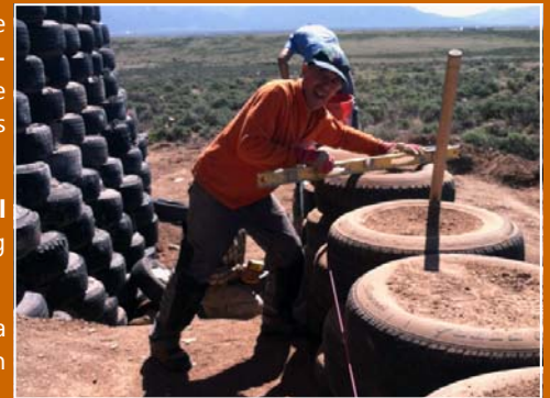
Leveling the rammed earth tire wall for the greenhouse (Taos)
