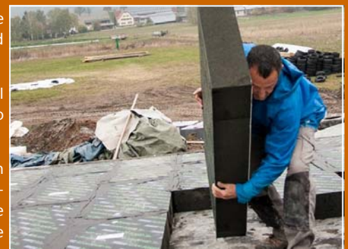
Recycled fiberglass panels for roof isolation (Tempelhof)
