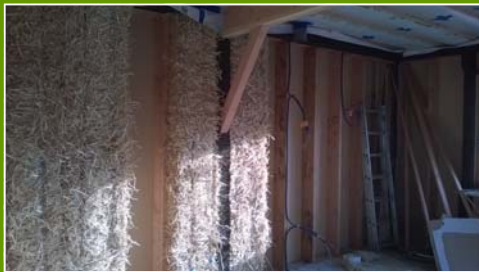
Straw, cork and vapor barrier on the ceiling
