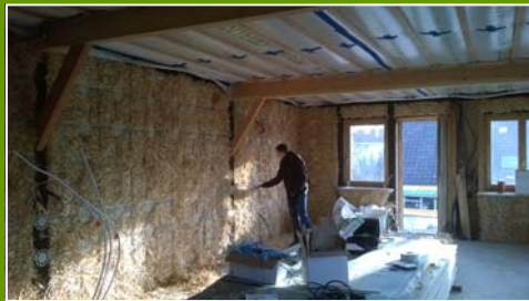
Laying the strips (interior)
