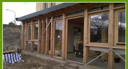
Wooden frame at the Montreuil site
