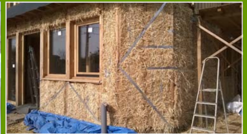
Laying the strips (exterior)
