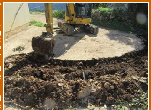
Decompacting soil that has been driven over for over 20 years
